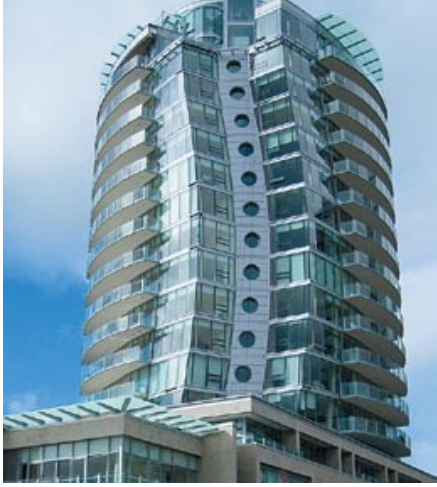
ULTIMATE LUXURY: Chambers Electric worked on the innovative Erickson project.
