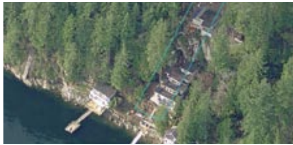
Left: High-tech photographic tools enable appraisers to view hard-to-access properties.
